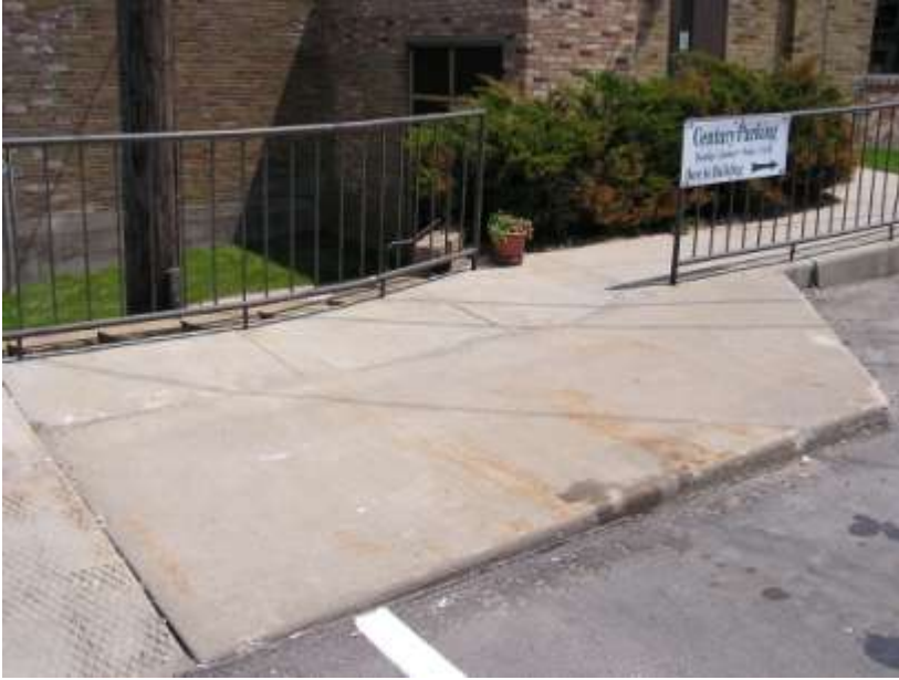
Sidewalk from Handicapped Stall to back door Slight slope and uneven sidewalk Stairs are located left of the door, concern about their location relative to door opening
