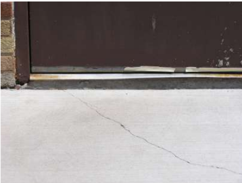
Back door – Concern about access to individuals in wheelchairs
